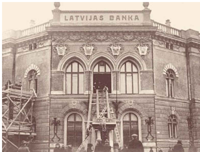
Lifting of the safe, 1920s. The works are managed by Pauls Tīlemanis, master locksmith of Riga. Following nationalisation, his workshop, located at Anglikāņu iela 3, was transferred to Latvijas Banka. The photograph was given to Latvijas Banka by the daughter of Pauls Tīlemanis on 10 August 1993.
